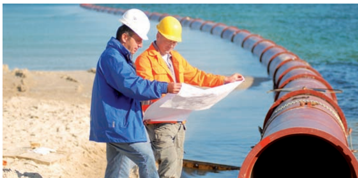
Floating in a ductile cast iron pipeline
