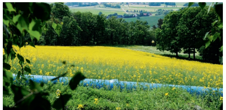
Temporary pipeline with BLS® joints
